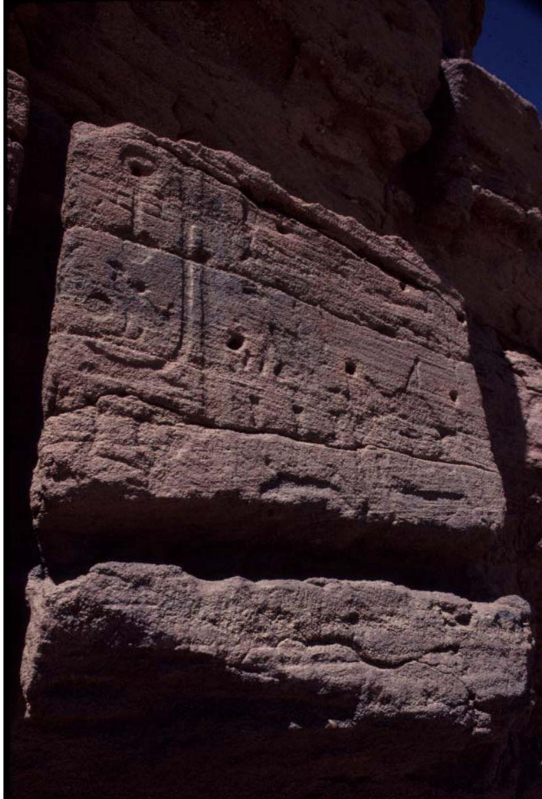
fig. 4. Panel with very worn texts of Taharqa, preserving rows of holes for nails, which had fastened gold sheet to the stone (See fig. 4). (Photo: T. Kendall)
