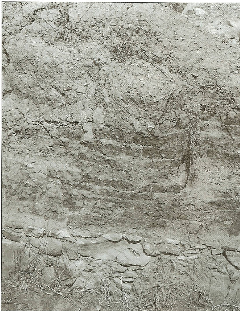
Individual sun-dried mud-bricks, which rest on a socle of rubble masonry, are clearly discernible in the West Gate of Eretria. As for the Athenians, the standard measurement employed by the Eretrians was the 'short foot'. (Author's collection)
