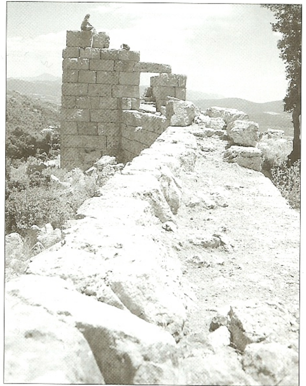
ABOVE Towers 2 to 5 have ground-floor chambers without loops or windows, and second chambers at parodos level with arrow slits. They were not, therefore, designed to house catapults but as battle-stations for archers. Tower 5 is seen here from Tower 4. (Author's collection)
