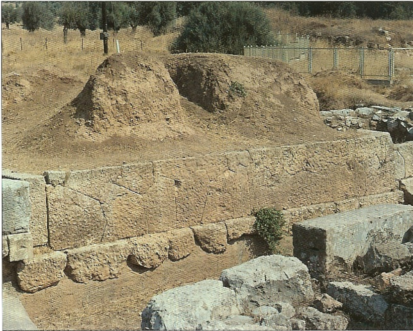
LEFT A common, cheap and effective building material, ancient mud-brick rarely survives today. Here we see 'melted' brickwork resting on a socle of 'Lesbian masonry', the North Tower of the West Gate, Eretria. (Author's collection)
