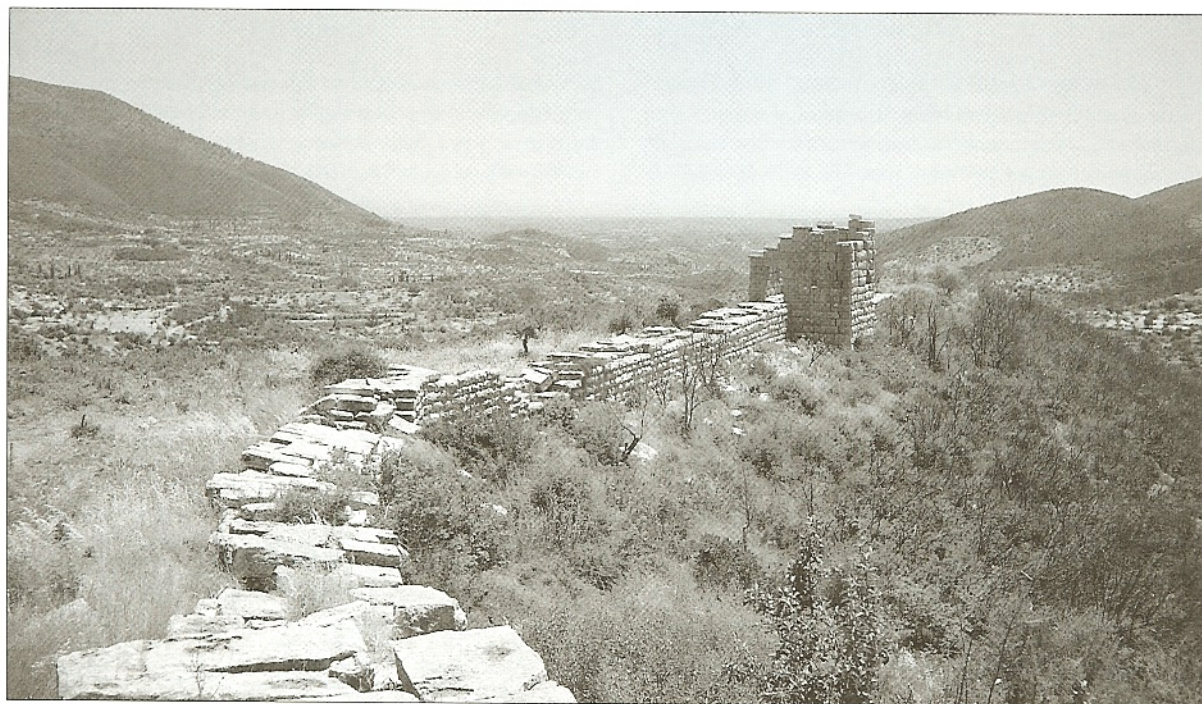
The west wall of Messene, looking south towards Tower N. This structure is an excellent example of a first-generation artillery tower. Built with a solid base, the tower consisted of a single chamber, housing non-torsion catapults, surmounted by a fighting-platform roof. (Author's collection)
